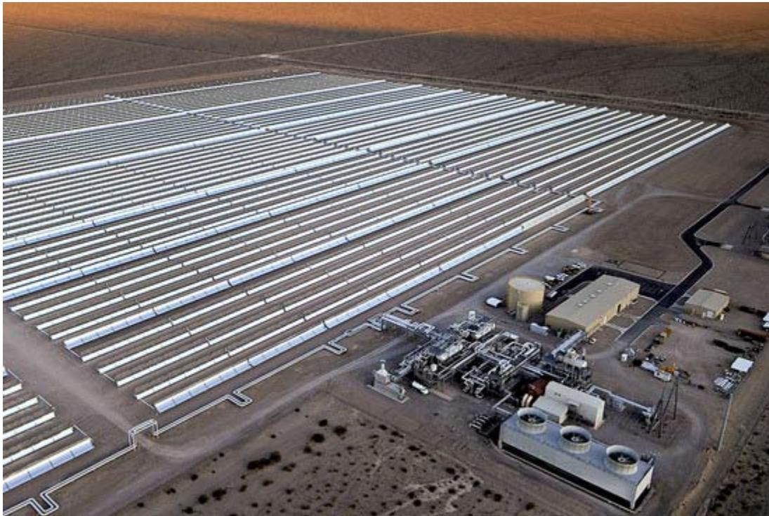
**THE TECHNOLOGY:** Energy from the sun can be used to make electricity directly with photovoltaic panels or indirectly using concentrated sunlight to heat a liquid, which produces steam to turn electrical
